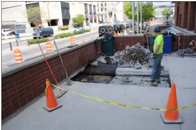
Blue Cross Arena West Terrace
